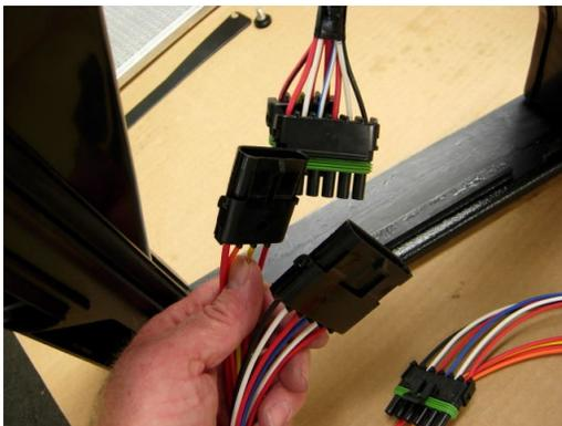
Clip the water tight connections together and push the wires back up into the return air side of the unit.
